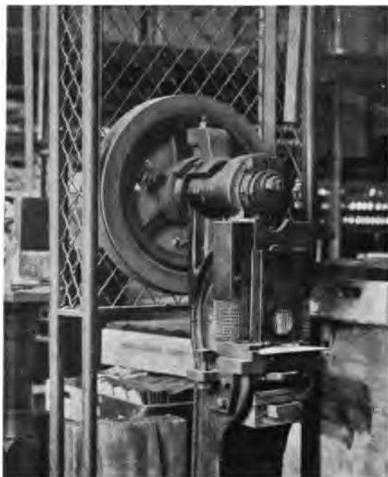
Fig. 1. Grill-Work Plunger-Guard.*
